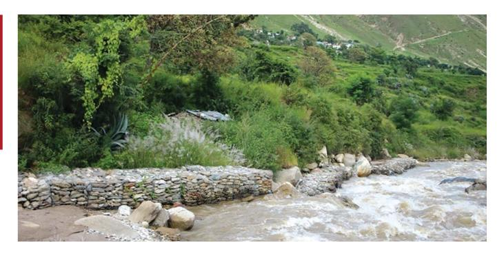
sixty thousand only). The result was the construction of 110-meterlong gabion protection wall that still provides protection to the village and their agricultural land!
